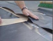
**Step 9**- Remove the release paper and allow the top PondGard panel to fall across the tape while pulling the release paper away at a 45° angle.
