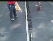
**Step 7**- Check the QuickSeam Splice Tape alignment to avoid "fish mouths" or folds in the tape.
