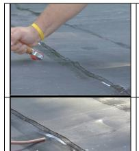
**Step 11**- Using a hand or stand-up roller; roll the seam longitudinally and across the seam in overlapping sections to mate the seam together.
