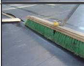
**Step 10**- Use a broom to brush over the splice to solidify the adhesion.
