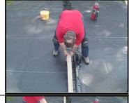
**Step 6**- Adhere the 3" QuickSeam Splice Tape to the primed surface of the bottom PondGard panel.
